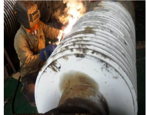
Crusher roll arcing
